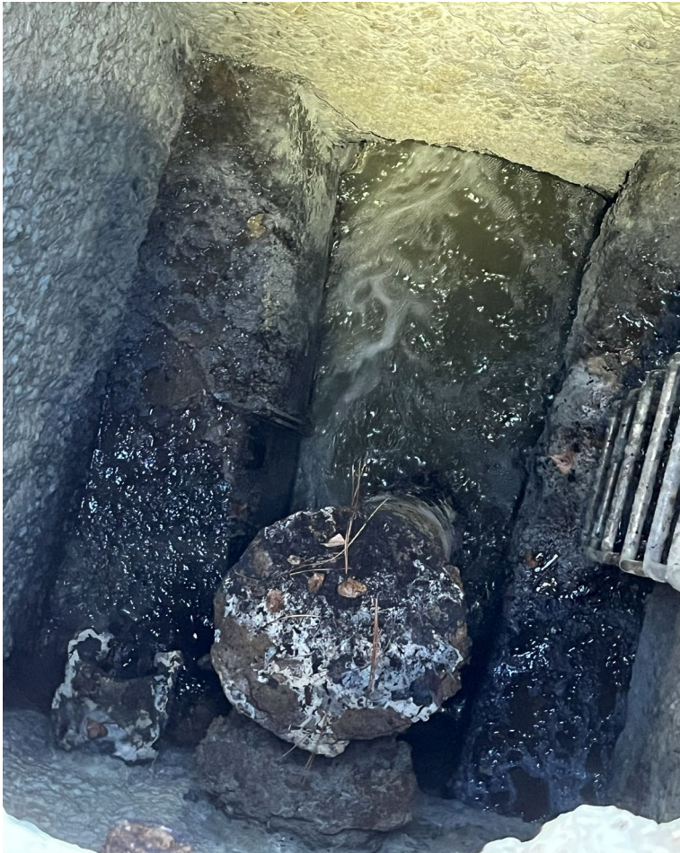
Found Condition – Major Corrosion
