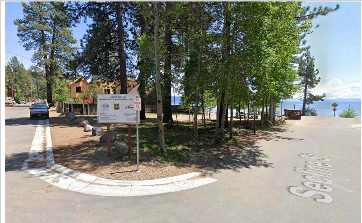
7. View to southeast from Secline Street/Brockway Vista Drive intersection towards the Concept B restroom structure location.
