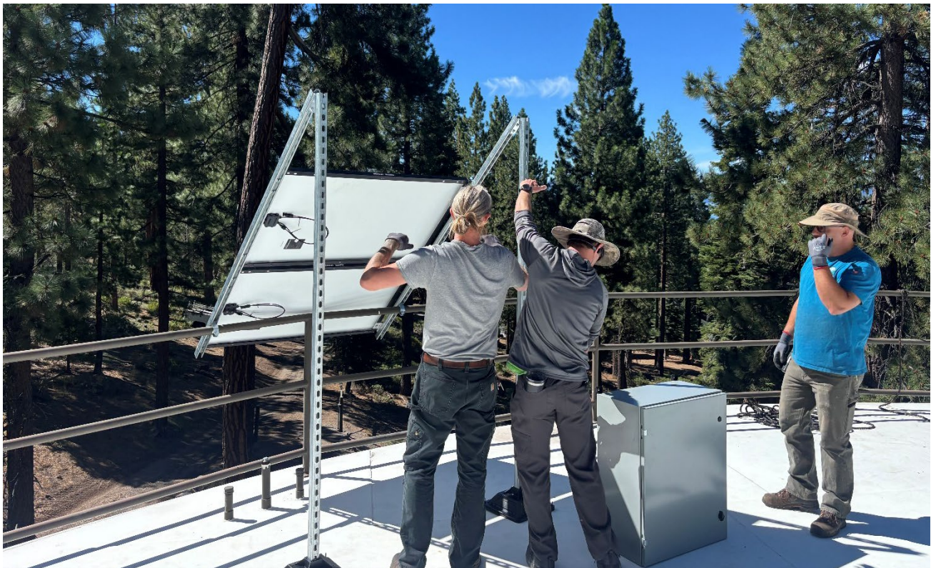
Crew installing a new solar panel on the Kings Beach Water Storage Tank.
