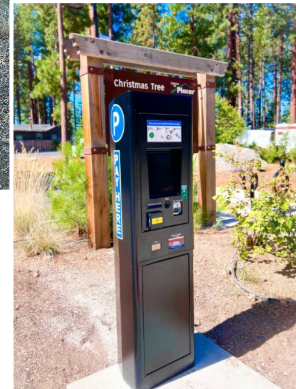
Installed Kiosk in Kings Beach
