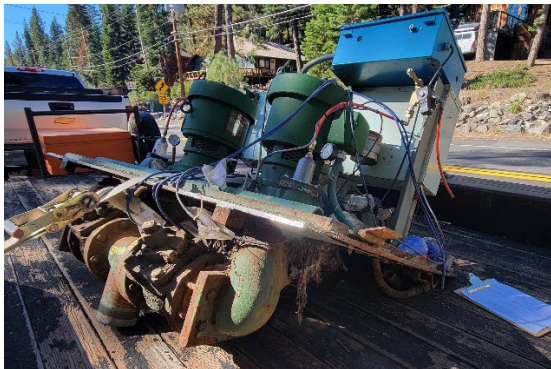
Old Pump Station D-5
