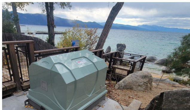
New station at S-1
