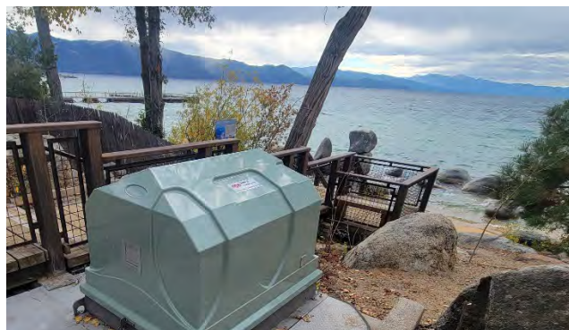
New station at S-1
