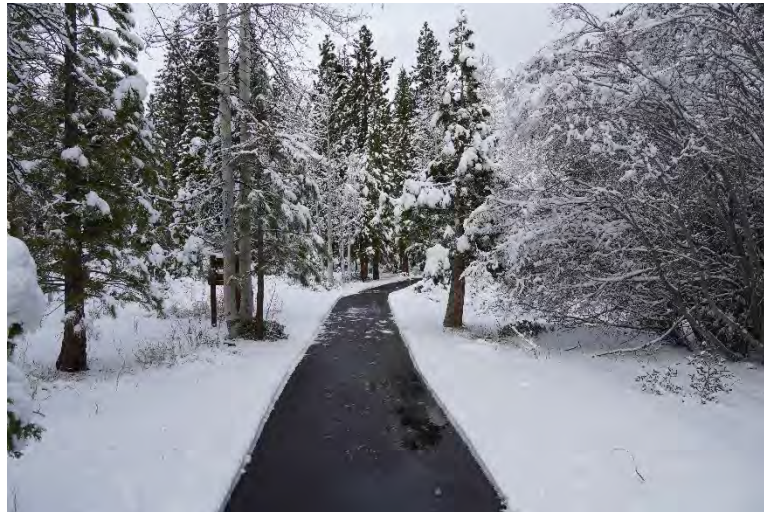
Clearing the Aspen ADA path with the Multi-Hog
