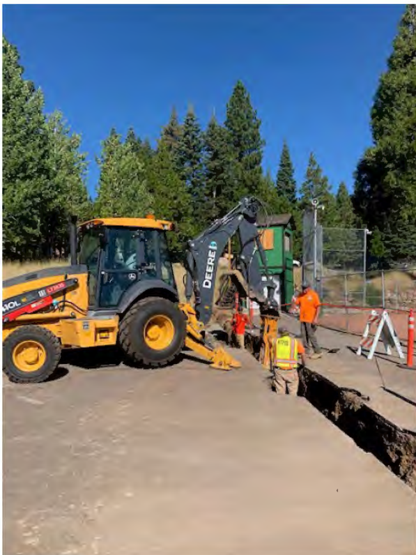
Conduit trench in the park at Ballfield #1 to bring power to the park entrance kiosk.
