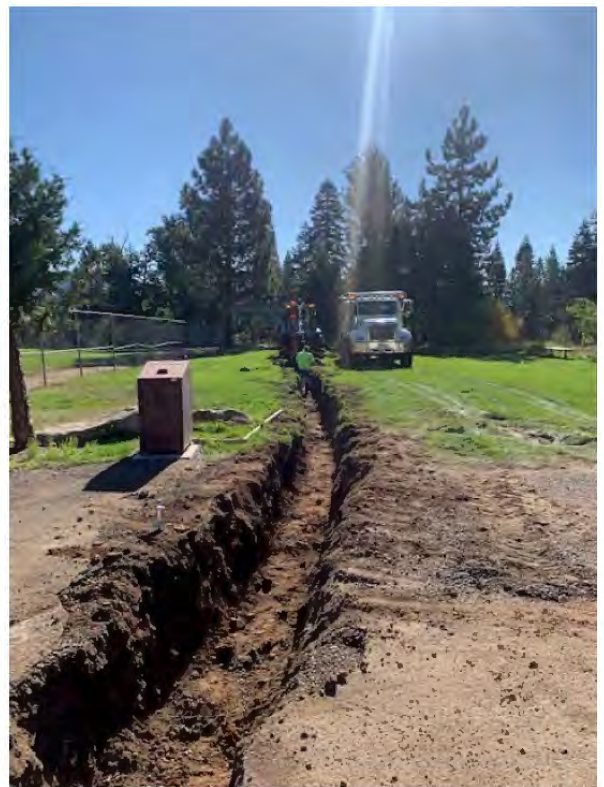
Conduit trench in the park at Ballfield #1 to bring power to the park entrance kiosk.
