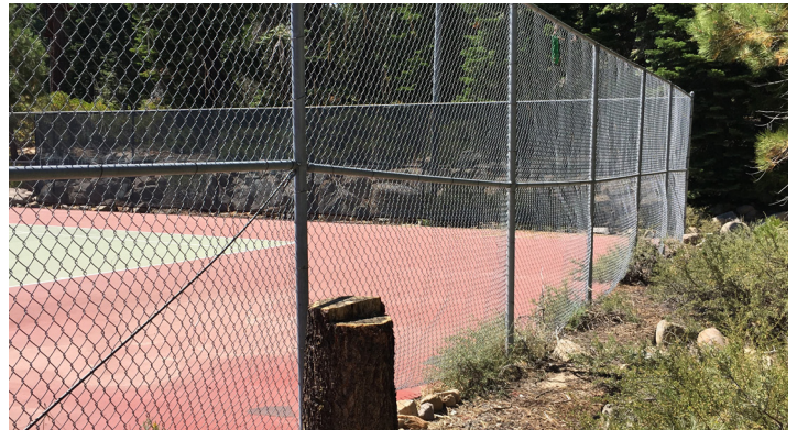
Image 8: Perimeter fence conditions
