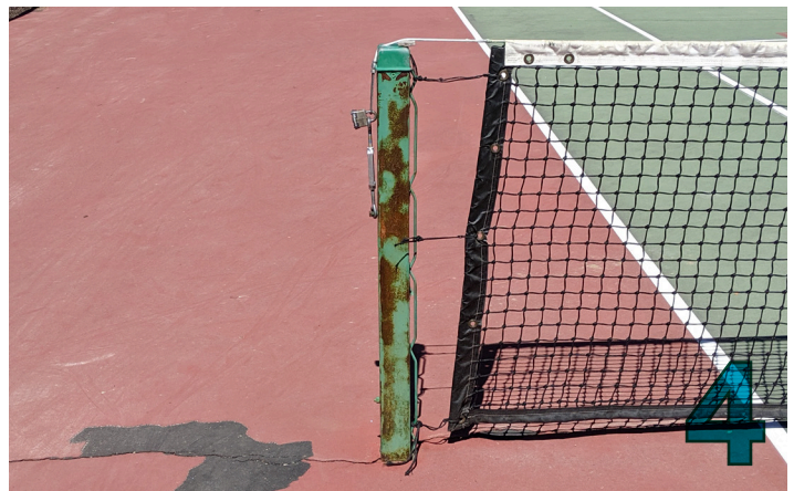
Court Furnishings in Disrepair
