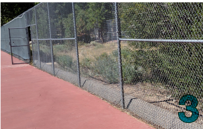
Perimeter Fence and Edge Conditions
