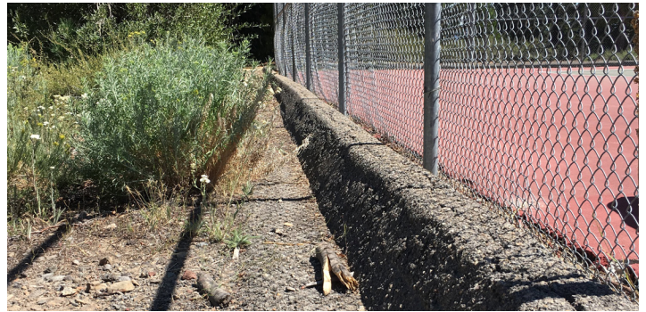
Image 10: Perimeter access curb
