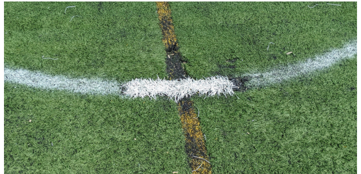
Image 6: Turf degradation and patching of turf
