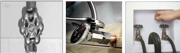
**Don't wait for an emergency.** Always know how to shut off the water supply to your entire house, or parts of it. Knowing the location of a simple shut-off valve could save thousands of dollars in damage. Everyone in your house should know where the valves are located and the direction they need to be turned to stop the flow.
