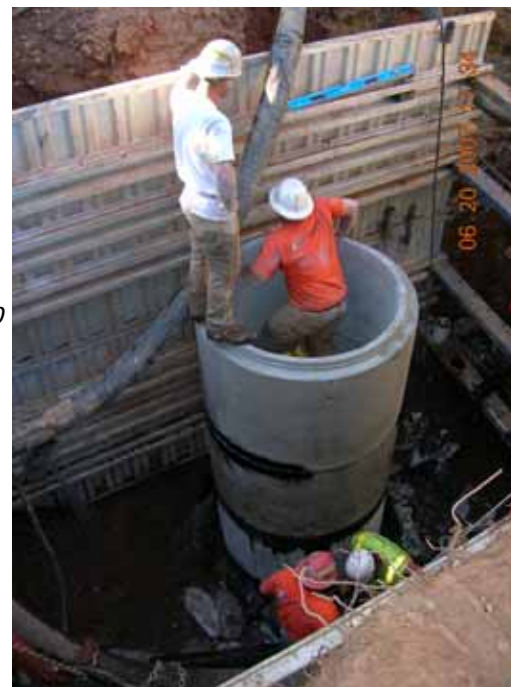
Installation of a new sewer line and manhole on Bay Street.
