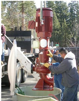
Installation of a new grinder pump at the Carnelian Main Sewer Pump Station. The pump uses mechanical cutters to chop debris that can and has caused clogging of sewer station pumps.
