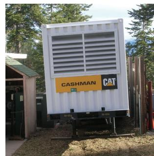
Emergency generator at the Dollar Lift Station. The District rented a backup generator to provide additional power in the event of commercial power disruption during high flow events for the winter months.
